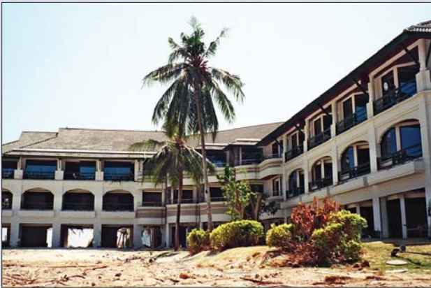
The damage to this modern beach hotel on Phi Phi Don Island in Thailand was limited to non-structural elements and contents
